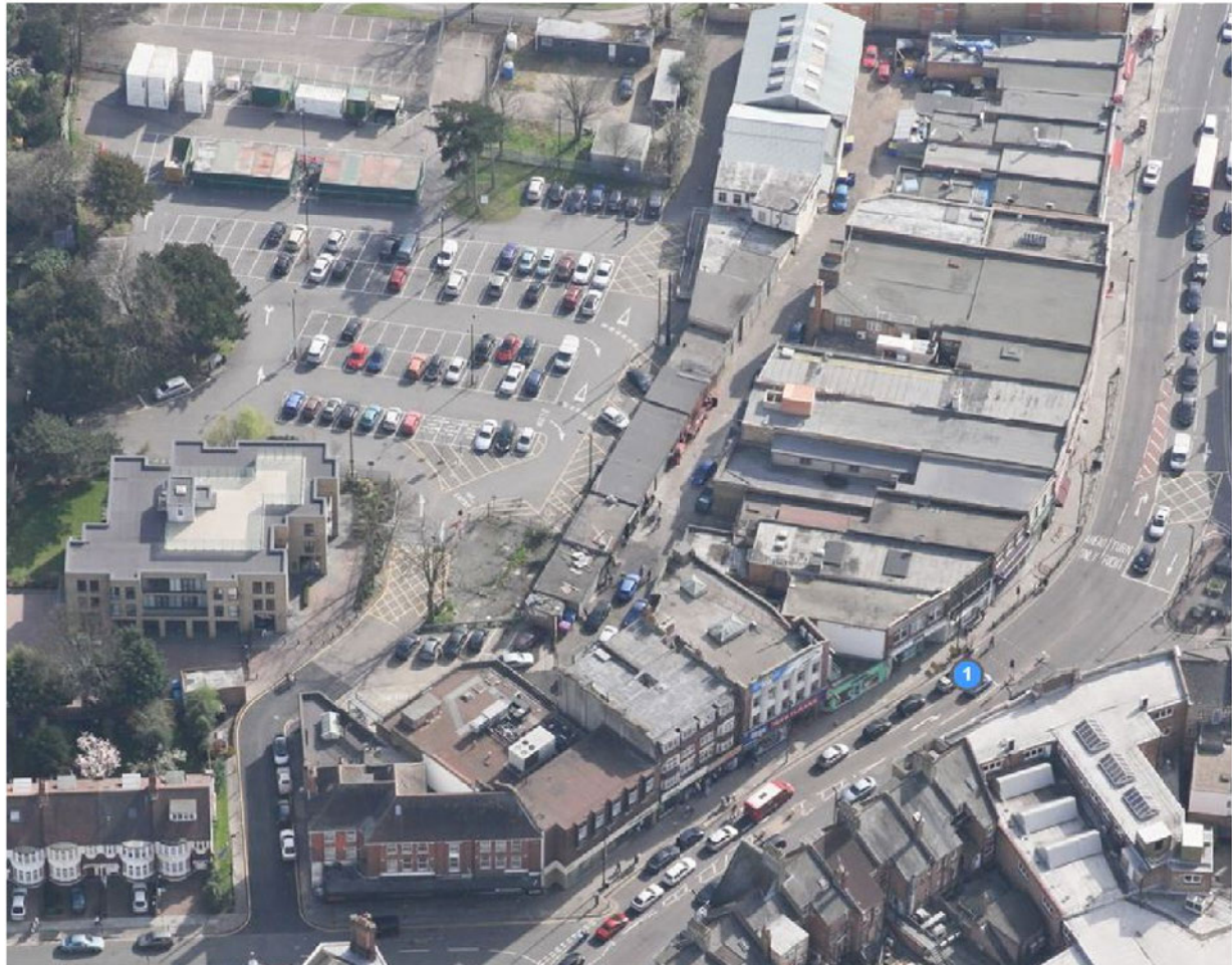
View to South
